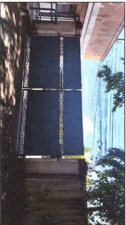
EXISTING ENTRANCE/EXIT VEHICLE GATE NOTE: FOR REPAIR AND REPAINTING
